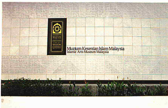
Main façade of the Islamic Arts Museum Malaysia with marble panels of Kufi Banaie script.
